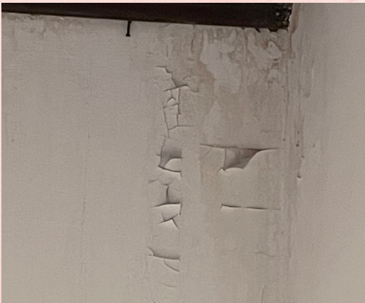
Water intrusion causing paint peeling & bubbling
